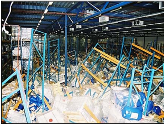
Image 11: collapse storage rack
